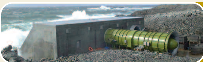
< The 500 kW Islay LIMPET Wave Power Plant has been successfully supplying energy to the electrical grid in the UK since November 2000.
